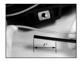
6.5 Snap the 3M<sup>TM</sup> FibrTube into the intended splice tray entrance location. Cut the FibrTube near the end of the retainer slot.
