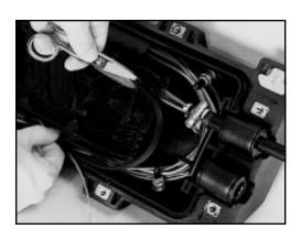
6.6 Remove the FibrTube and unzip it by grasping and separating the two upper ridges.
